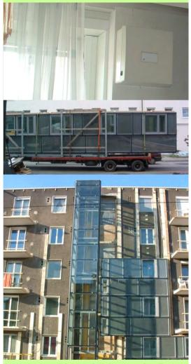
Prefabricated and mounted wall units
