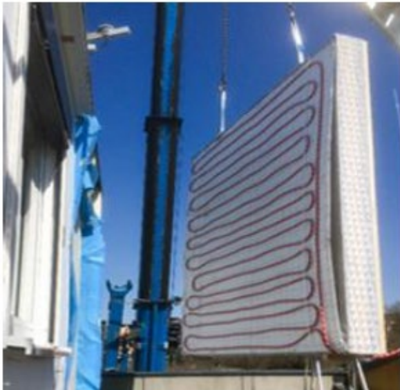
Figure 21: Velcro mounted heat dissipation system for building mass activation retrofit (left) and mounting of the prototype on the facade energy test rig at the laboratory of AEE INTEC (right), source AEE INTEC.
