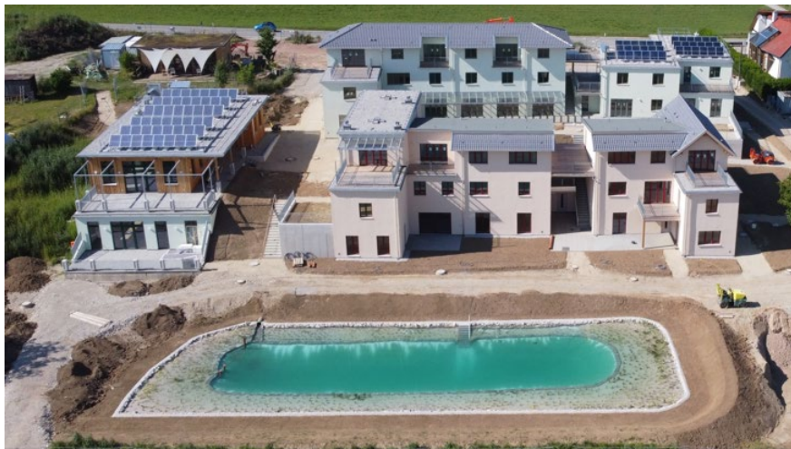
Figure 39: Concluded first building phase of the "Garten der Generationen" with solar thermal production units and a thermally utilizable pond as one part of multiple storage capacities in the system. [Source: Garten der Generationen e. V.]
