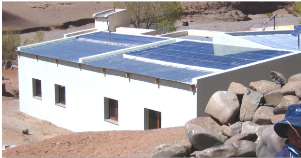
Solar air heaters and rock bed before filling at primary school in Misa Rumi/Altiplano/Argentina [2]
