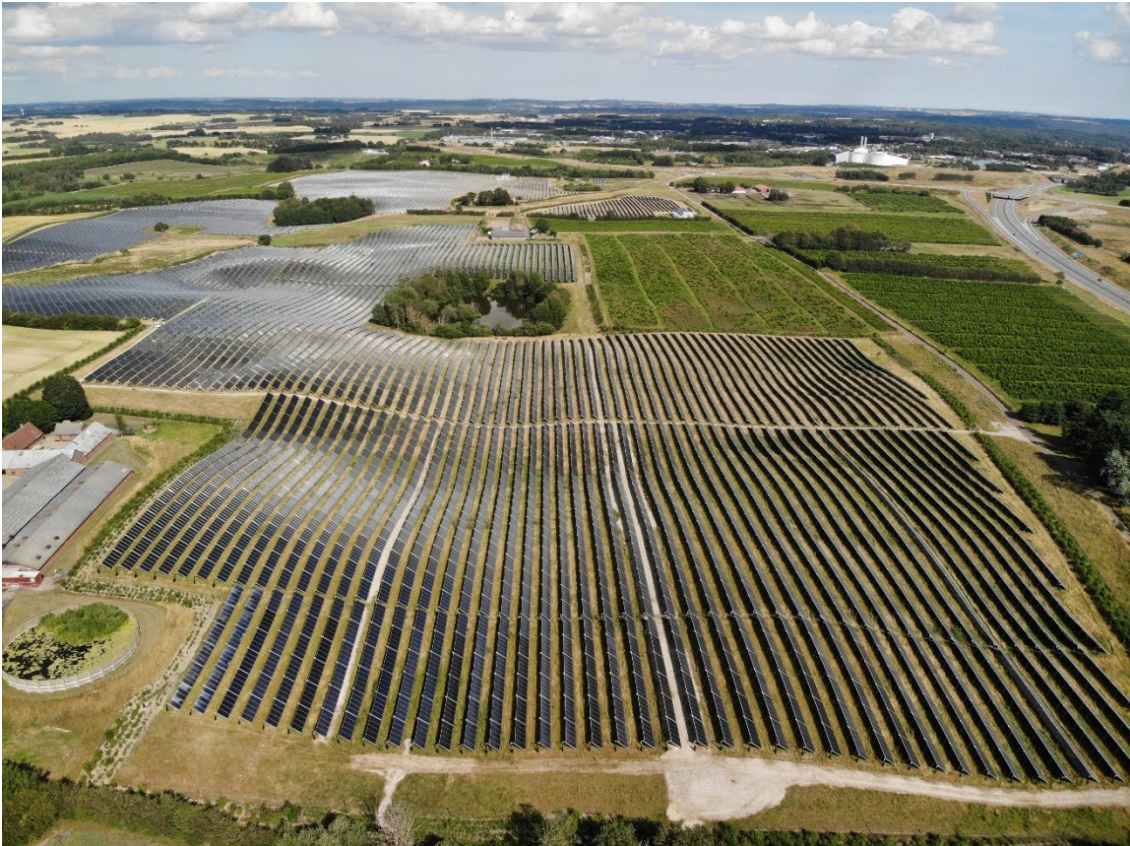
Solar collector field with a total collector aperture area of 156,694 m 2 at Silkeborg solar heating plant. (DTU)
