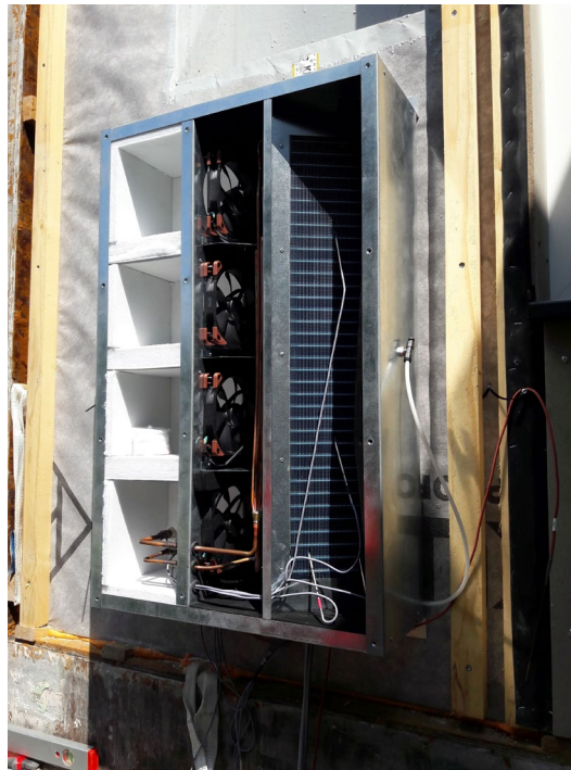
Outdoor unit of the developed mini-split air-to-water heat pump with open casing. The evaporator as well as the four axial fans are shown in the foreground. Sound absorbing panels (in white) were employed on the outflow to minimize sound emissions. (Source: Monteleone et al., 2024)
