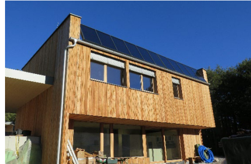
Figure 25: South view of a solar house in Tyrol (picture source: Building Owner)
