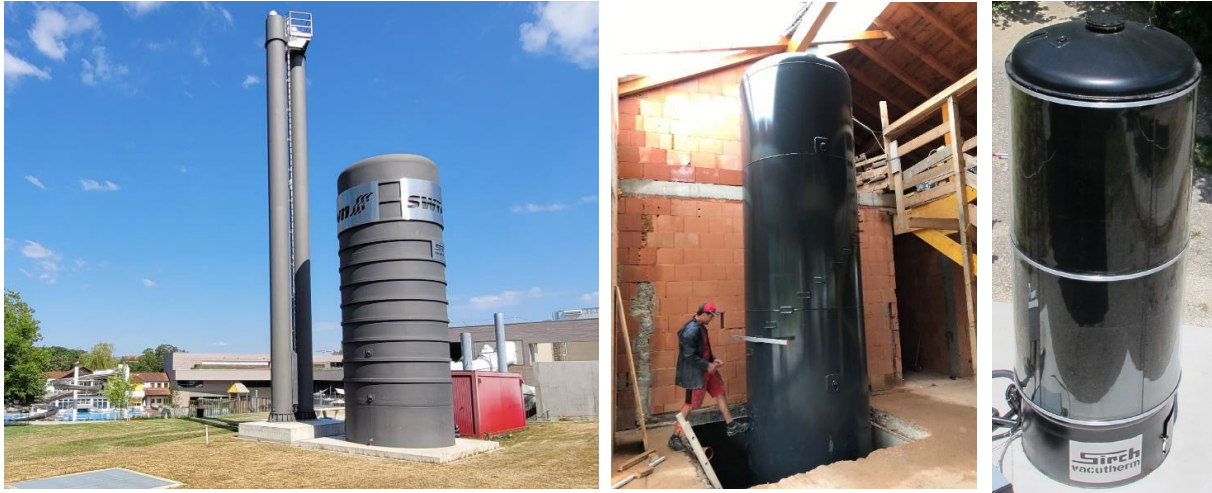
Double-walled vacuum insulated hot water stores by the manufacturer Sirch. Left: hot water store with 60 m 3 water volume, installed at a public pool in Neumarkt (Germany), driven by combined heat and power plants (CHP); middle: hot water store with 8 m 3 water volume, installed inside a new-built private dwelling in Kirchdorf (Austria); right: hot water store with 12 m 3 water volume and additional transparent thermal insulation (glass), installed at an outdoor test rig of the Institute for Building Energetics, Thermotechnology and Energy Storage (IGTE) of the University of Stuttgart. Pictures made by IGTE.
