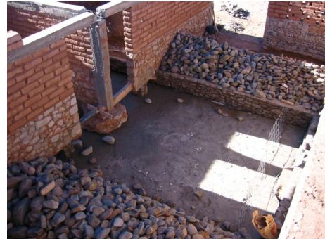
Solar air heaters and rock bed before filling at primary school in Misa Rumi/Altiplano/Argentina [2]
