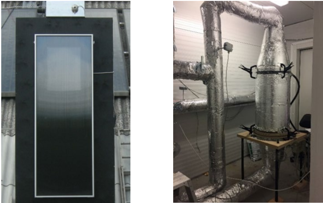
Figure 3 Example: Air solar dehumidifier (Solarventi, Andersen, 2011) (left) Cold storage and ventilation duct system (Nielsen, E., Becker-Hardt, S., Englmaier, S., Kong, W., Furbo, S., 2022) (right)
