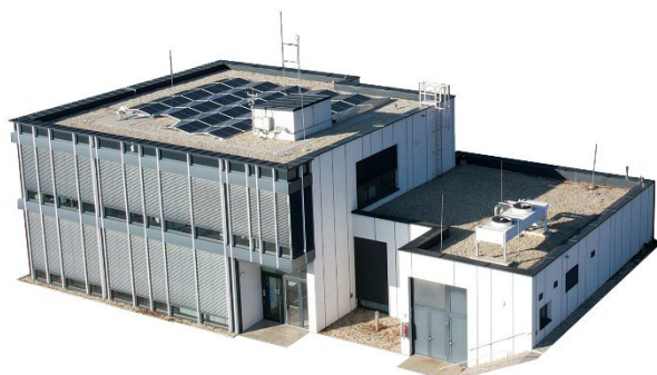
Energetikum Office Building
