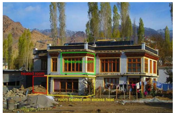
Figure 3: Schematic of heating system and Kurja Guest house with solar air heater on roof
