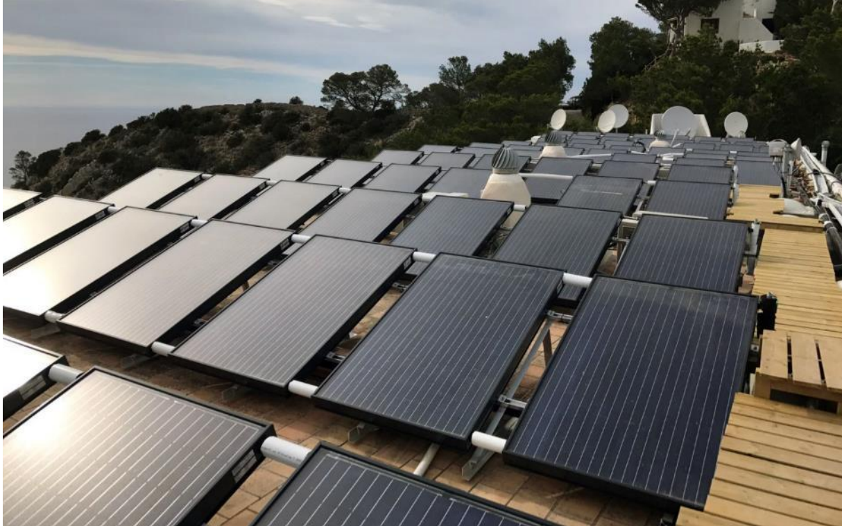
Figure 11: View of the PVT solar installation on the roof of a luxury hotel in Ibiza.
