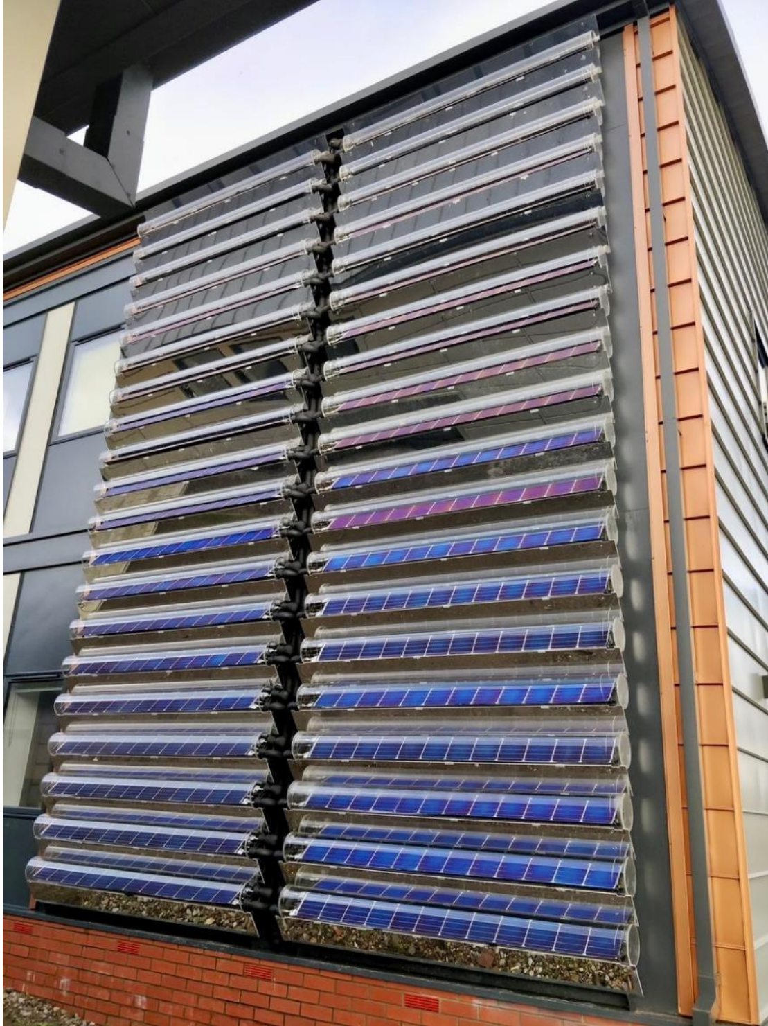
Figure 50: The evacuated tube PVT array (Virtu PVT by Naked Energy) on the south facing façade of the Active Office building at the University of Swansea.
