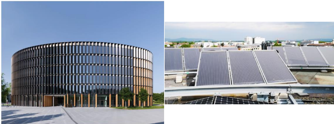
Figure 32: View of the new town hall with façade-integrated PV modules (© Stadt Freiburg) and the PVT collector array on the roof (© Manuel Lämmle).
