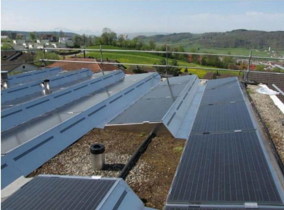
Figure 40: View of the PVT system on the roof of the single-family house in Wettswil.
