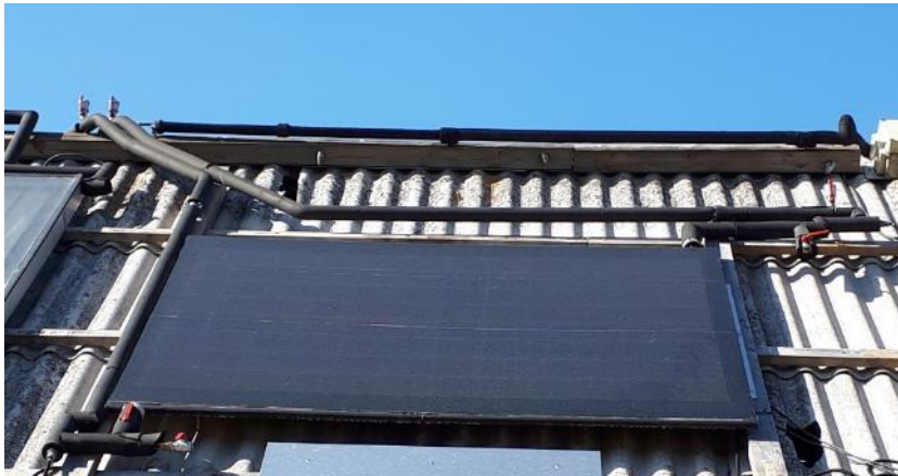
Figure 56: View of the PVT collector on the test facility at DTU.
