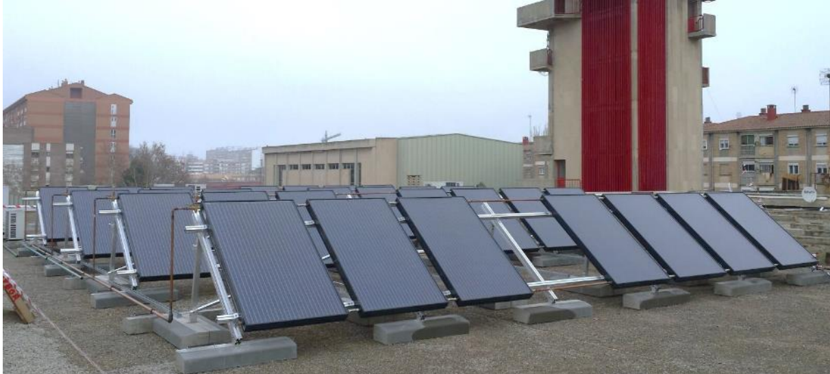
Figure 13: View of the PVT field in firefighters building.
