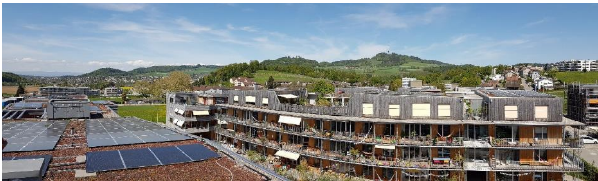
Figure 37 : View of the building B (background) in front part of the PVT system on the roof of building C
