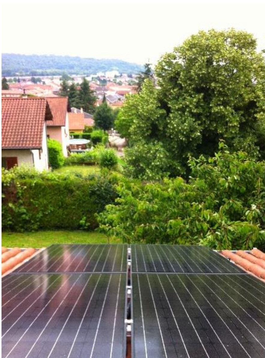
Figure 24: View of the PVT system on the roof of the single-family house in Ambérieu.
