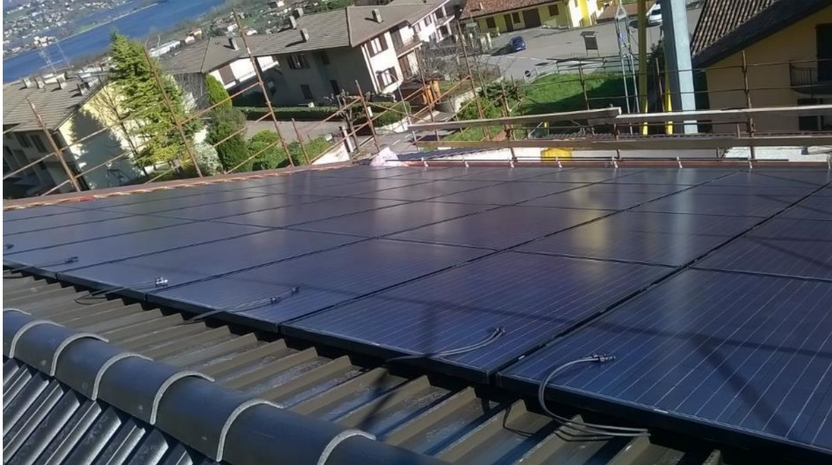
Figure 35: View of the PVT system on the roof of the single-family house in Suello (Lecco).
