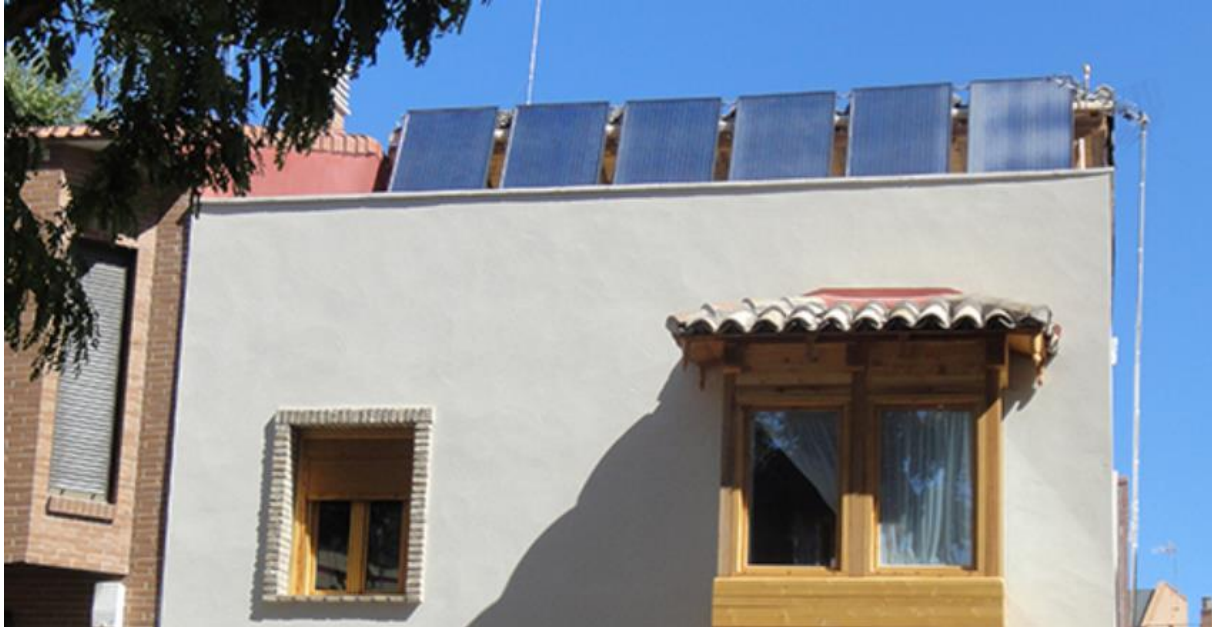
Figure 9: View of the 6-PVT solar installation in single family house.
