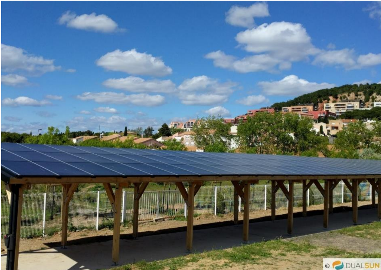
Figure 28: View of the PVT canopy for the municipal swimming pool in Sète
