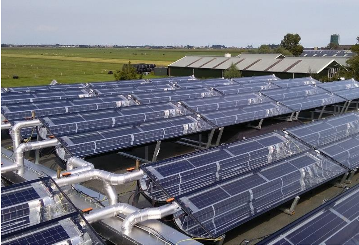
Figure 52: View of the PVT system on the roof of Henri Willig cheese factory in Katwoude, the Netherlands.
