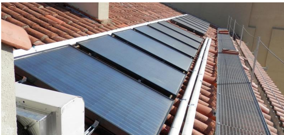
Figure 7: View of the roof-mounting PVT installation in the urban centre of Zaragoza.
