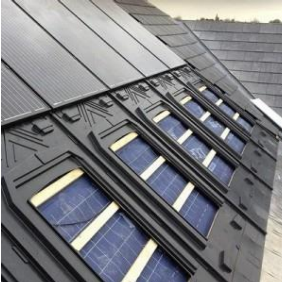
Figure 46: View of the PVT air system on the roof.
