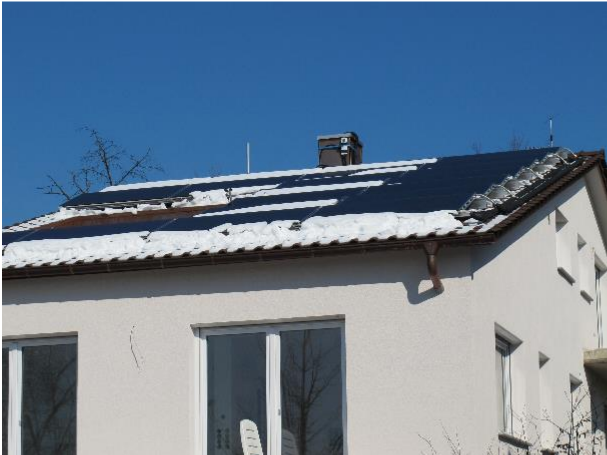
Figure 44: View of the PVT field on the single family house in winter.
