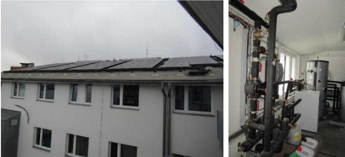
Figure 34: PVT system on the roof of the multi-family house (left) and technical room with ground source heat pump and storages (right)
