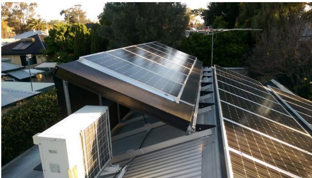
Figure 48: View of the PVT system on the roof of the single story family house in Perth.
