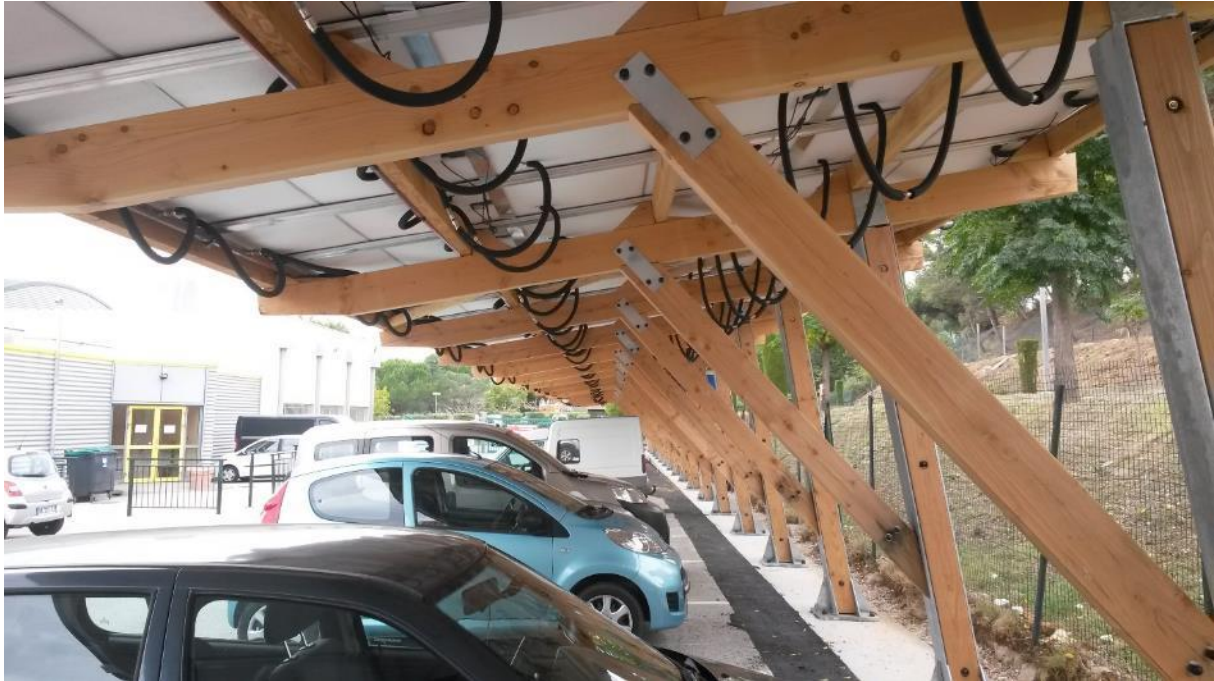
Figure 30: View of the PVT canopy for the municipal swimming pool in Perpignan
