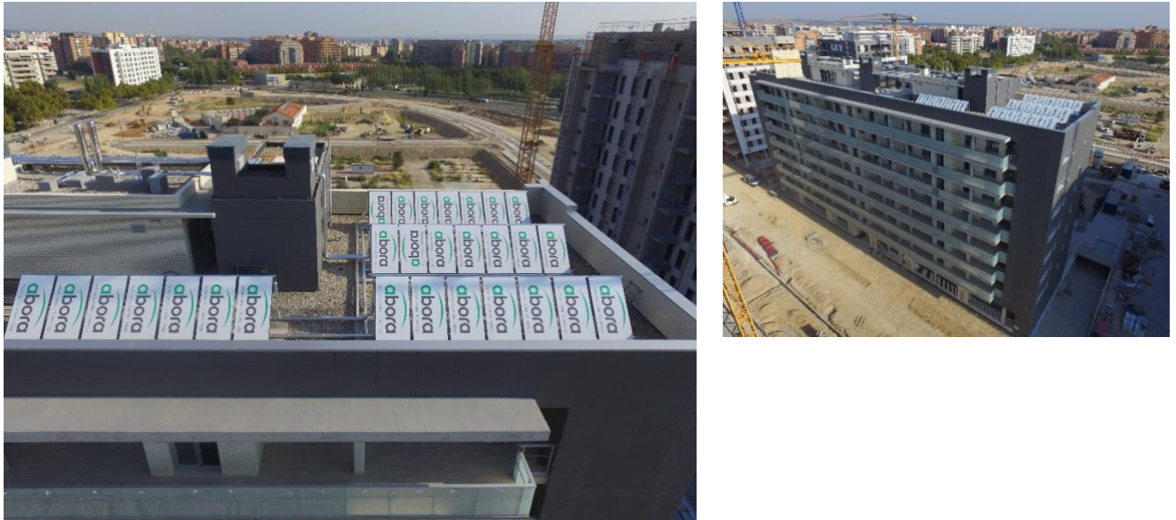
Figure 22: View of the PVT panels “Multi dwelling Azud”.
