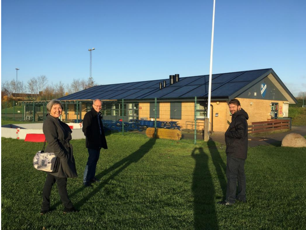
Figure 42: View of the BIPVT system integrated in the roof of the football club house in Stenloese
