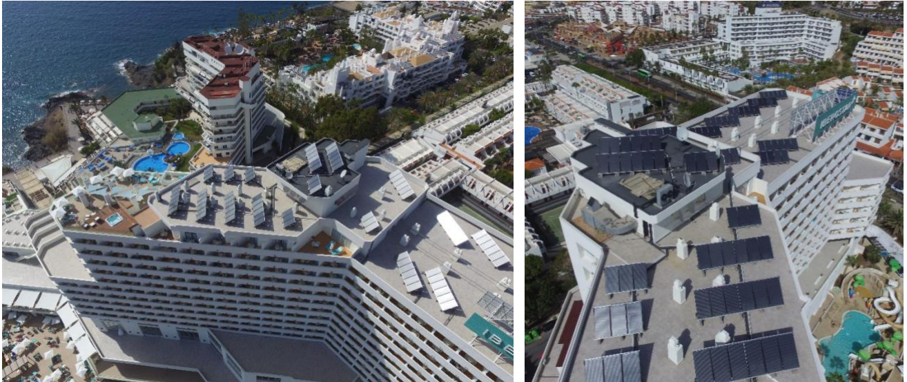
Figure 17: View of PVT in the flat roofs of Hotel Iberostar Buganvilles
