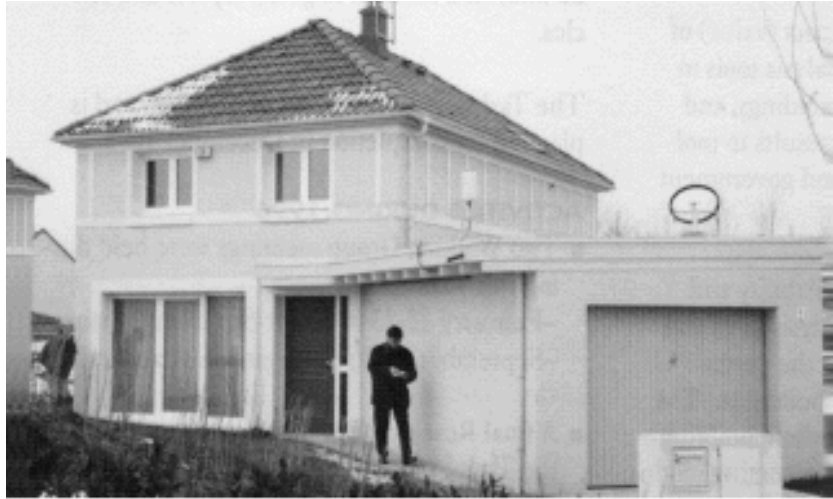
Exterior view of one of the two Lisses Test Houses operated by Electricity of France in Lisses, France
