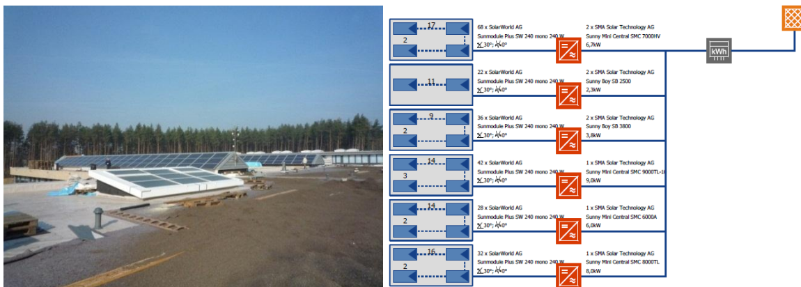
Figure 26: Roof with PV system and roof light (left); Screenshot of the PV system planned with PV*Sol (right).
