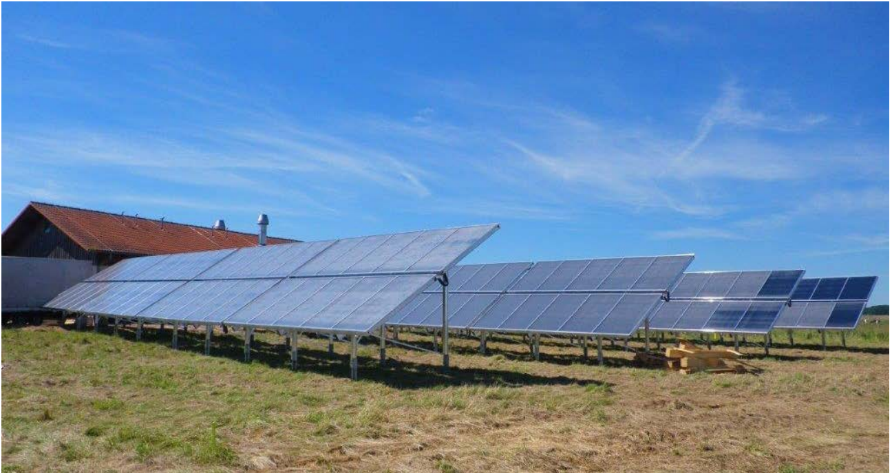
Figure 1: Field of flat plate collectors close to the GPRS building (Source: Enersolve)
