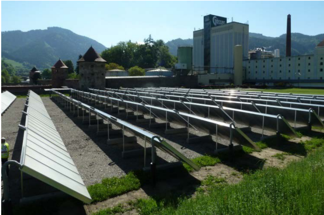
Figure 6: Flat-plate collector field with 1,500 m 2 at the Goess Brewery (Source: AEE INTEC)
