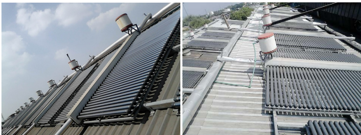
Figure 9: Evacuated tube collectors on the roof of Wheels India in Padi, Chennai, with a collector gross area of 1,365m 2 (Source: IEA SHC Task49 & SoPro India)
