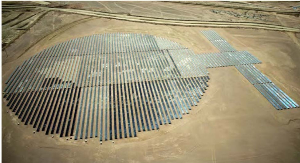
Figure 12: Flat-plate collector field of 39,300 m 2 at Codelco's "Minera Gabriela Mistral" in the Atacama Desert, Chile (Source: ArconSunmark)
