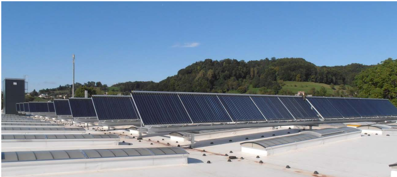
Figure 13: Field of 80 high performance evacuated tube collectors with CPC reflectors on the roof of Zehnder in Gränichen, Switzerland, with a gross area of 394 m 2 (Source: Ritter XL Solar)
