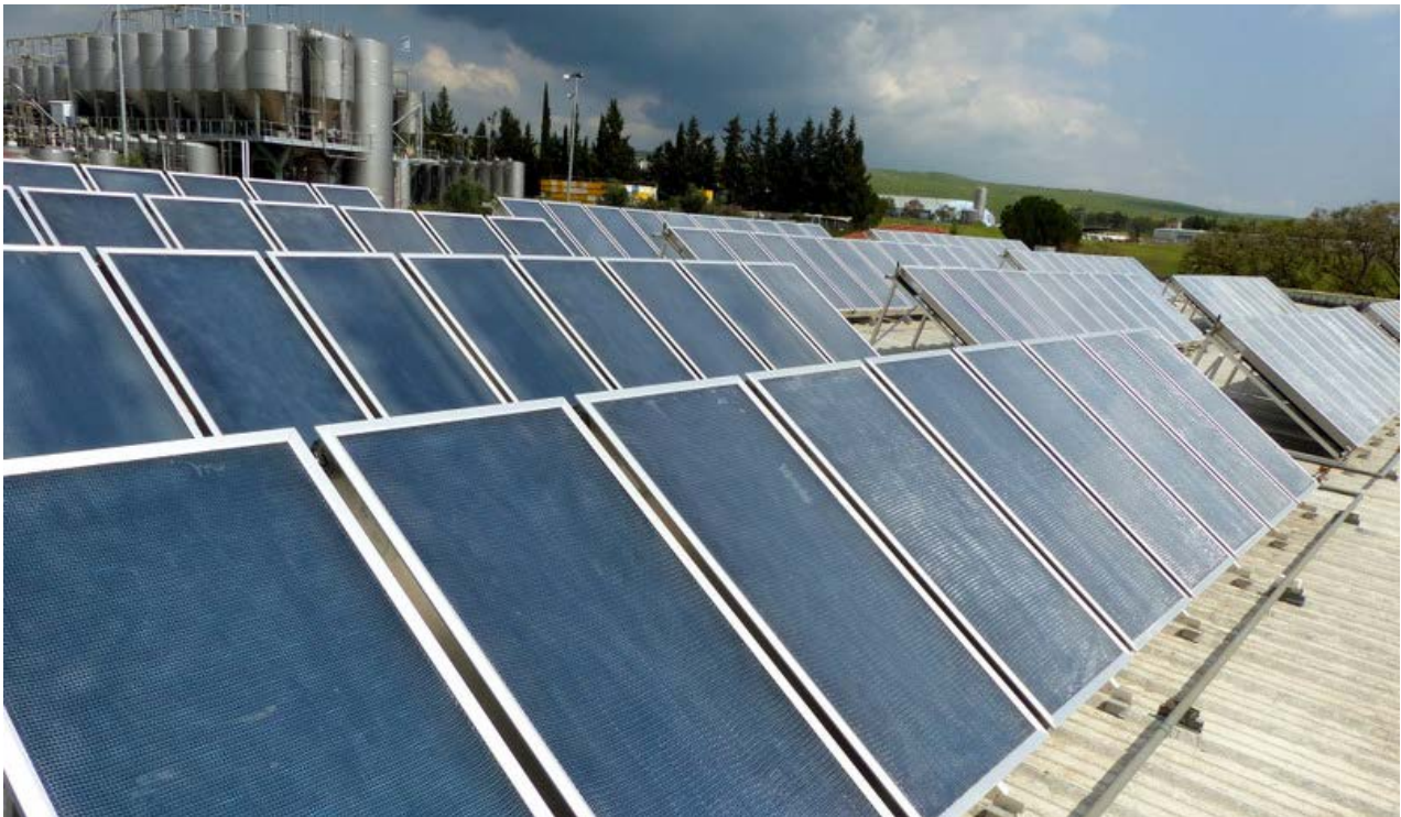
Figure 3: roof mounted solar system at Golan Winery (Source: TIGI Limited)
