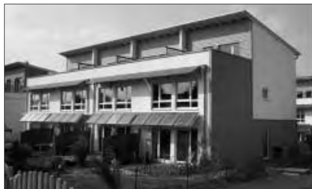
Figure 2a. Demonstration project in Gelsenkirchen, Germany. Source: C. Petersdorff, ECOFYS, Germany
