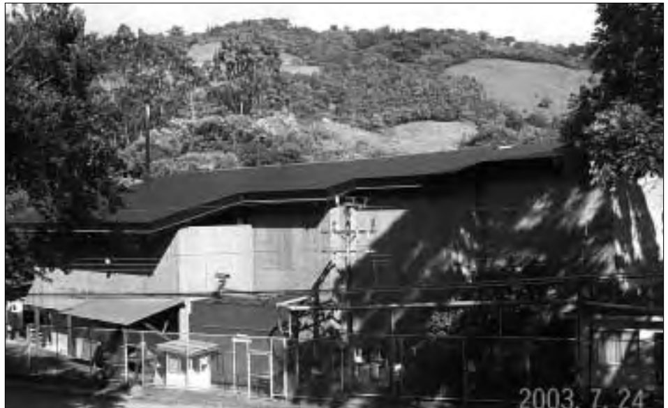
A solar system was installed on an existing coffee drying facility in the western mountains of Costa Rica. The system is expected to be commissioned in time for this year's harvest season.
