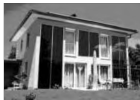
Solar combisystem with 22.7 m 2 façade-integrated collector in Austria
