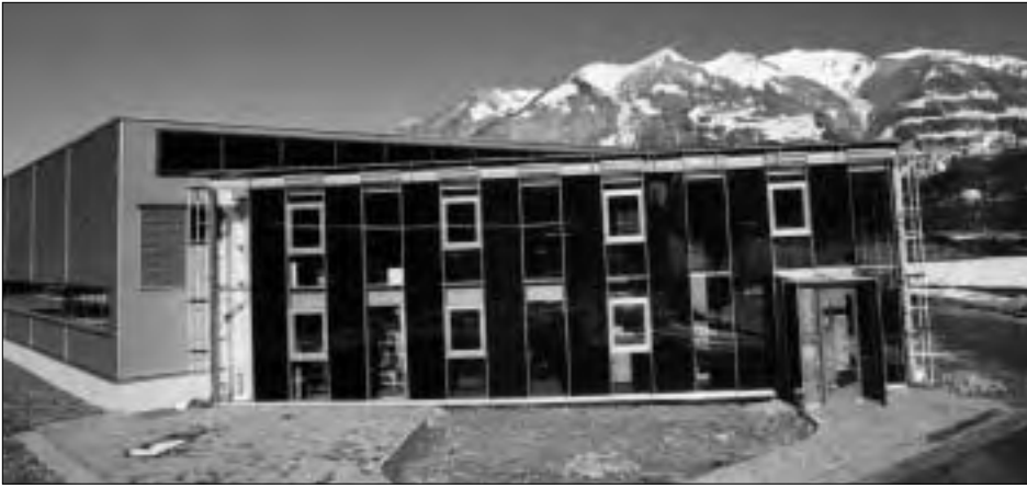
This production hall in Bludesch, Austria uses a flat plate collector (87 m 2 ) for space heating. The operating temperature is 20 - 80°C. Source: AEE INTEC, Austria
