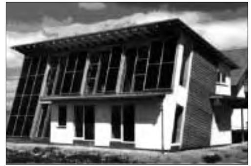
Solar Combisystem with facade-integrated collector array in Germany.
