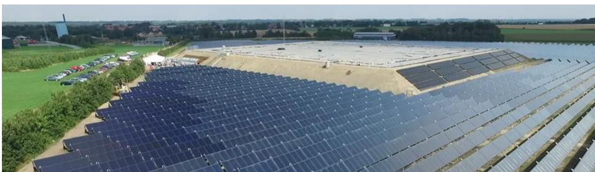
Figure 9 : The solar district heating system in Gram with damvarmelager [<http://www.gram-fjernvarme.dk/>]
