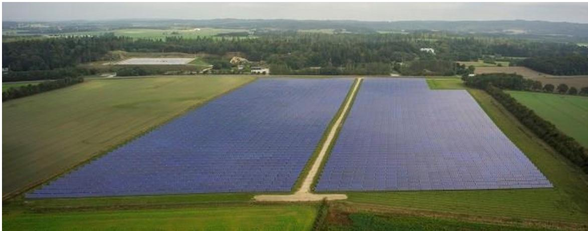
Figure 10 The solar district heating system is 37,573 m<sup>2</sup> with a pit heat storage of 60,000 m<sup>3</sup>. Dronninglund District heating is described here: <http://www.drlund-fjernvarme.dk/>, also a brochure can be found here.
